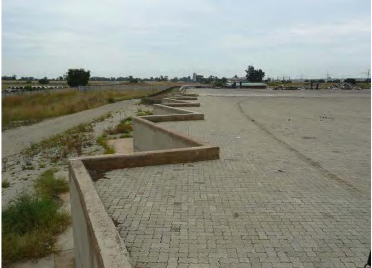
Orkney Transfer Station-Ramp method
